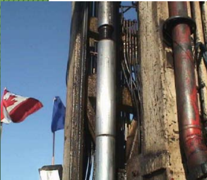
Pulling Out Mud Motor
